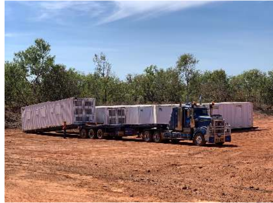
ACCOMMODATION UNITS BEING UNLOADED ON SITE AT LEGUNE
